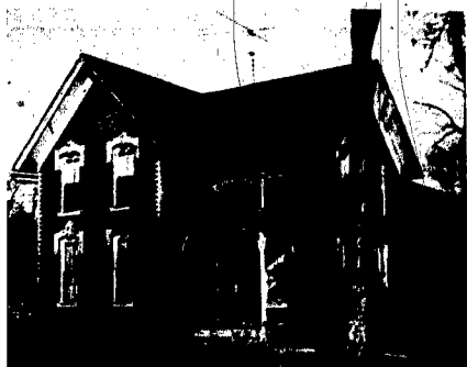
TO BE DISMANTLED soon is the 83 year old Wayne County jail and sheriff's residence. Built four years prior to the construction of the Court House in 1899 the brick building is scheduled for demolition this fall.
