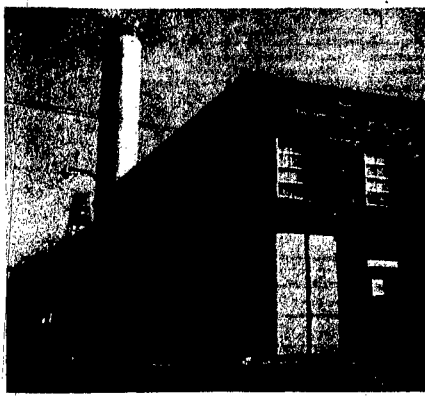
WAKEFIELD NATIONAL BANK has been undergoing extensive remodeling both inside and out during the past month. The remodeling contract was given to Structural Design Inc. of Iowa. When finished the building will feature new lighting, heating, air conditioning, more lobby area, a sound proof room for computing machines, and an additional business window.
